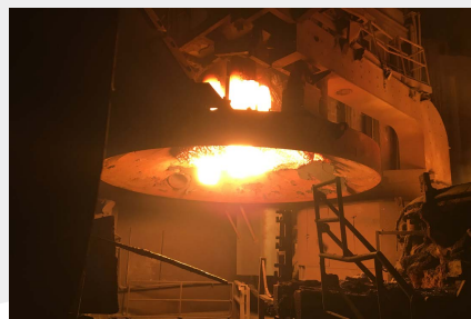
Bottom view of the roof after several heats showing less skulls compared with previous roof design
